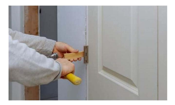
When your door doesn't close properly and leaves visible gaps between the door and the frame, it's a sign of a misaligned door frame. You can rectify this issue by adjusting the hinges or shimming the door frame. First, try tightening or loosening the screws on the hinges to align the door better. If that doesn't work, insert wooden shims between the door frame and the wall to adjust the positioning. Ensure that the door is level and plumb before securing the shims in place. Once
