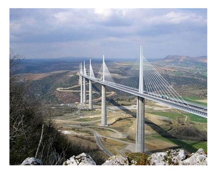
Considered a marvel of modern engineering, the Millau Viaduct in Southern France stretches across the Tarn Valley. This cable-stayed bridge holds the record for being the tallest bridge in the world, with its highest pillar reaching a height of 343 meters. Designed by renowned architect Norman Foster, this bridge not only serves as a vital transportation link but also showcases the endless possibilities of human imagination and engineering ingenuity.
